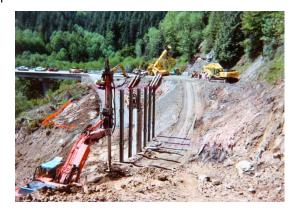
SR 508 is a two lane highway hung on the side of the mountain as it curves thru Bear Canyon. The overburden, saturated with rain water from the November storm, slid down the 20 degree rock slope leaving the residents with a 25 mile detour.
