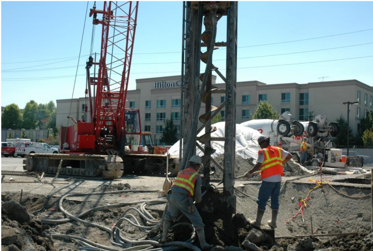
**Less noise** - Auger cast piles are a drilled and pumped pile, not a driven pile. This eliminates the hammer impact noise created by driving piles.
